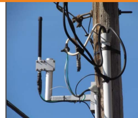
L BRACKET (Heavy Wall Hot Dipped Galvanized Steel Bracket)
